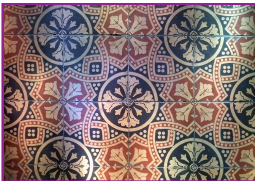
Chancel tiles from 1871
